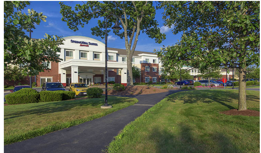
Marriott Spring Hill Suites (Connected to Conference Center via enclosed walkway)
